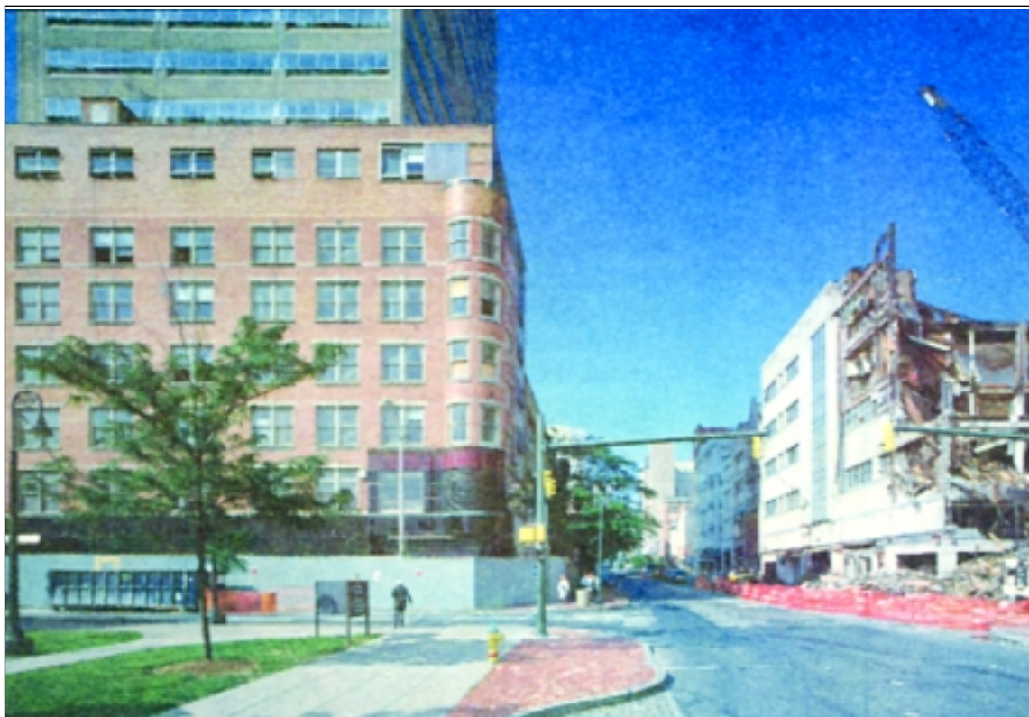
The Governor Hotel (left) has avoided the fate of the former Pomeroy's building in downtown Harrisburg. The old hotel is to be renovated by Progressive Investments, the only bidder which did not opt to tear it down.
